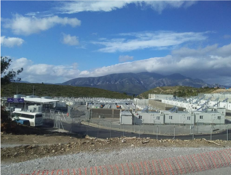
View of the new Closed and Controlled Access Centre (CCAS) on Samos Island. December 2021. Photo by Aideen Elliot
