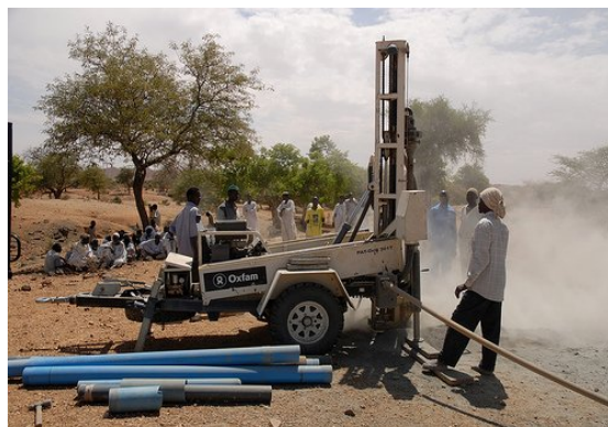
Drilling for water in North Darfur
