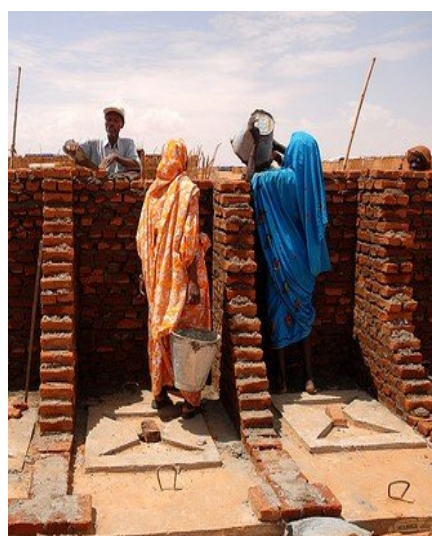
Constructing new latrines
